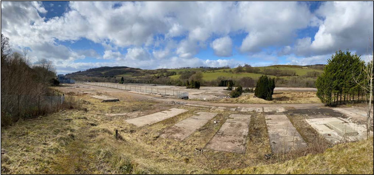
Looking west across the site from the path to the station
